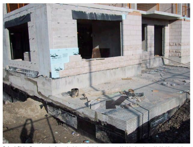
**Doing It Right** - Rare example of a condominium project where masonry block back-up is used behind the exterior insulation and brick facade. Note the use of punched windows instead of window wall assemblies from floor to ceiling. This type of construction provides superior durability and energy performance for a marginal premium.
