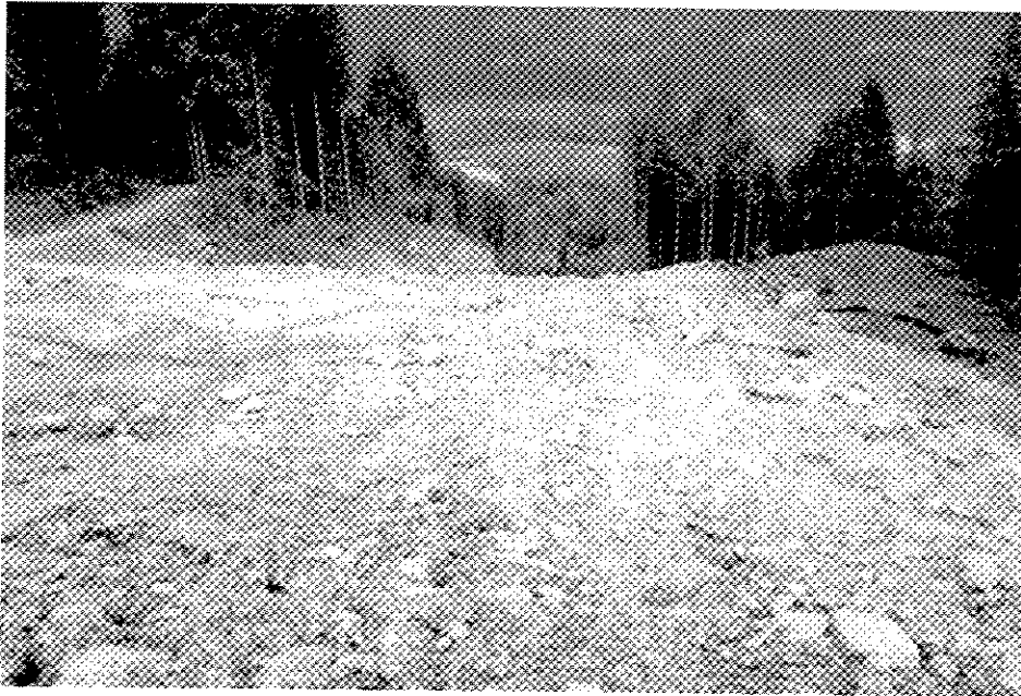
Figure 6. Penstock and access road clearing at Tipella.
